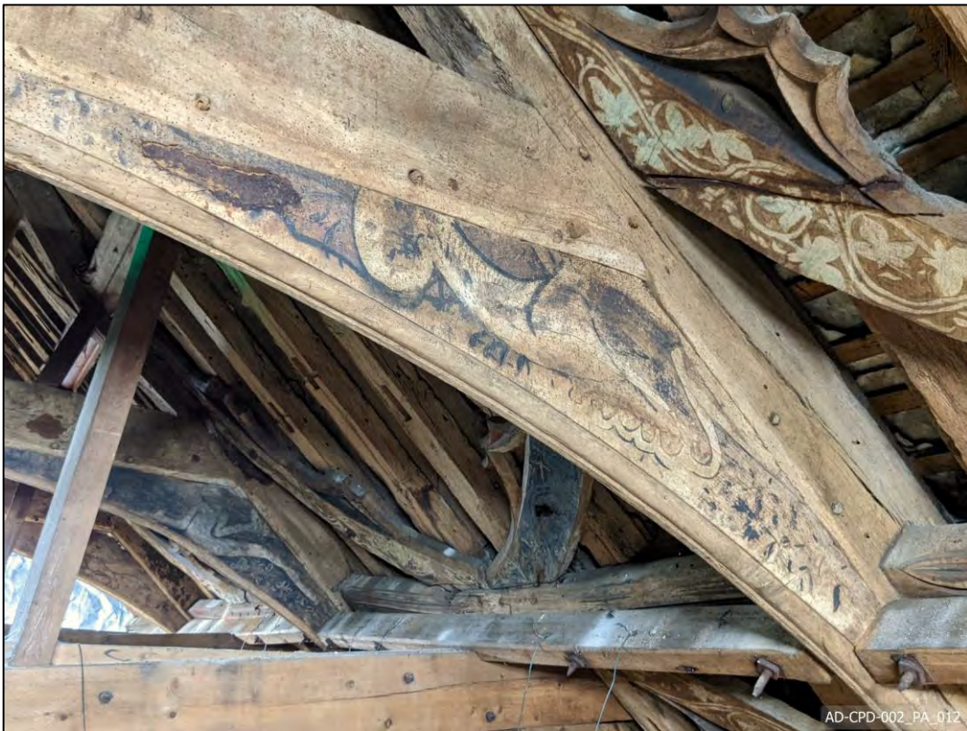
Plate 12 – Truss 8 – Painted Arch-brace – South
