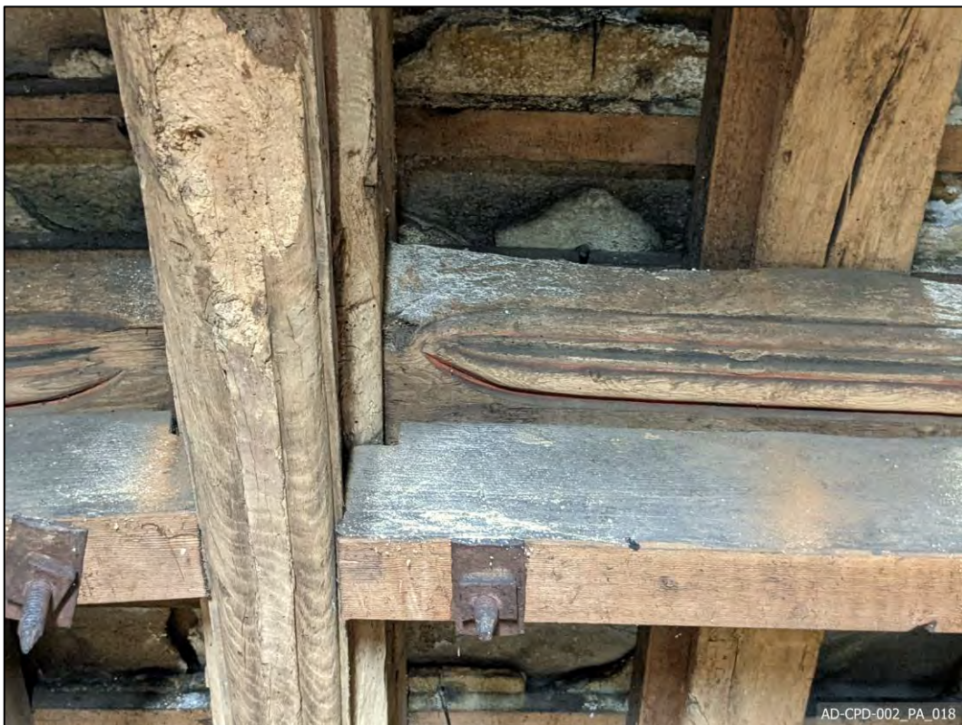
Plate 18 – General detail – Middle purlin
