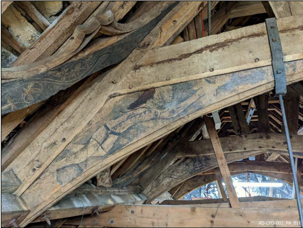
Plate 11 – Truss 8 – Painted Arch-brace – North
