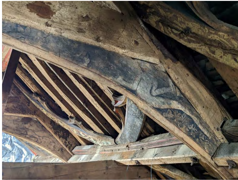
Fig. 1 – Painted Arch-Brace.
