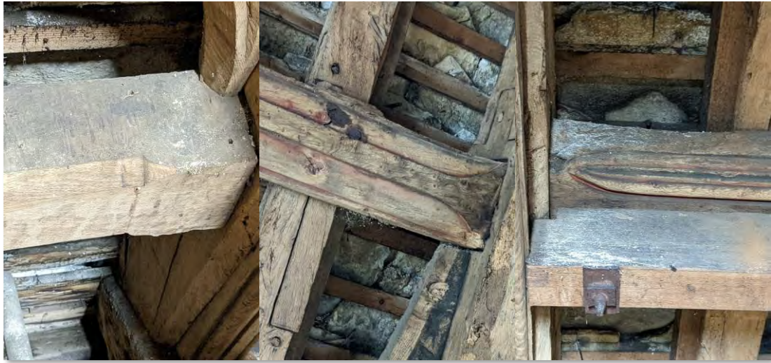
Fig. 6 – Chamfer and stop details
