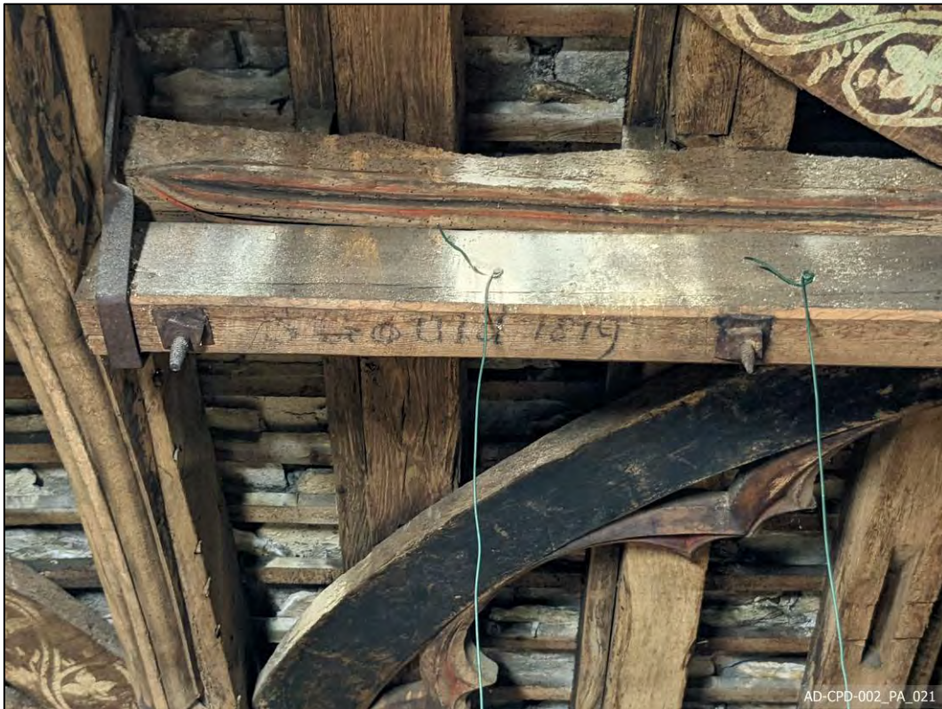
Plate 21 – Bay 4 – 1819 strengthening to purlin
