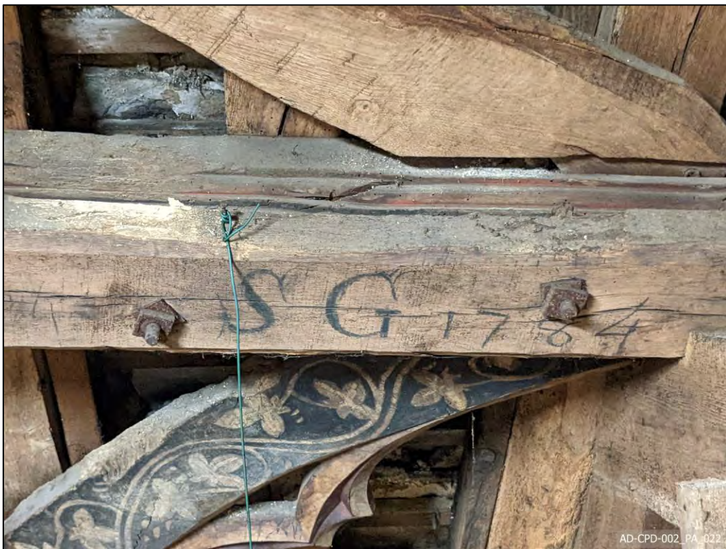
Plate 22 – Bay 13 – 1784 strengthening to purlin
