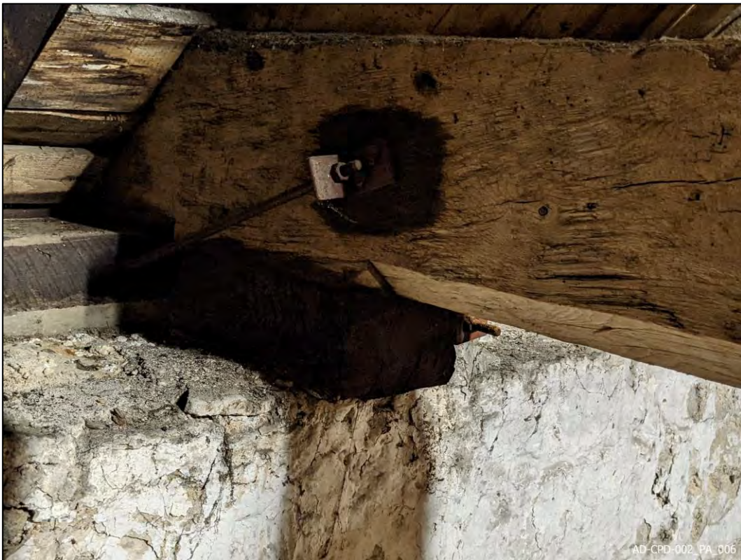
Plate 6 – Truss 2 – North – Tie-beam chamfer and stop
