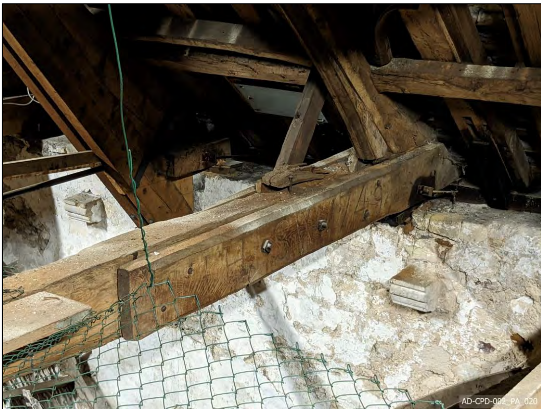
Plate 20 – Truss 9 – 1749 repair to tie-beam
