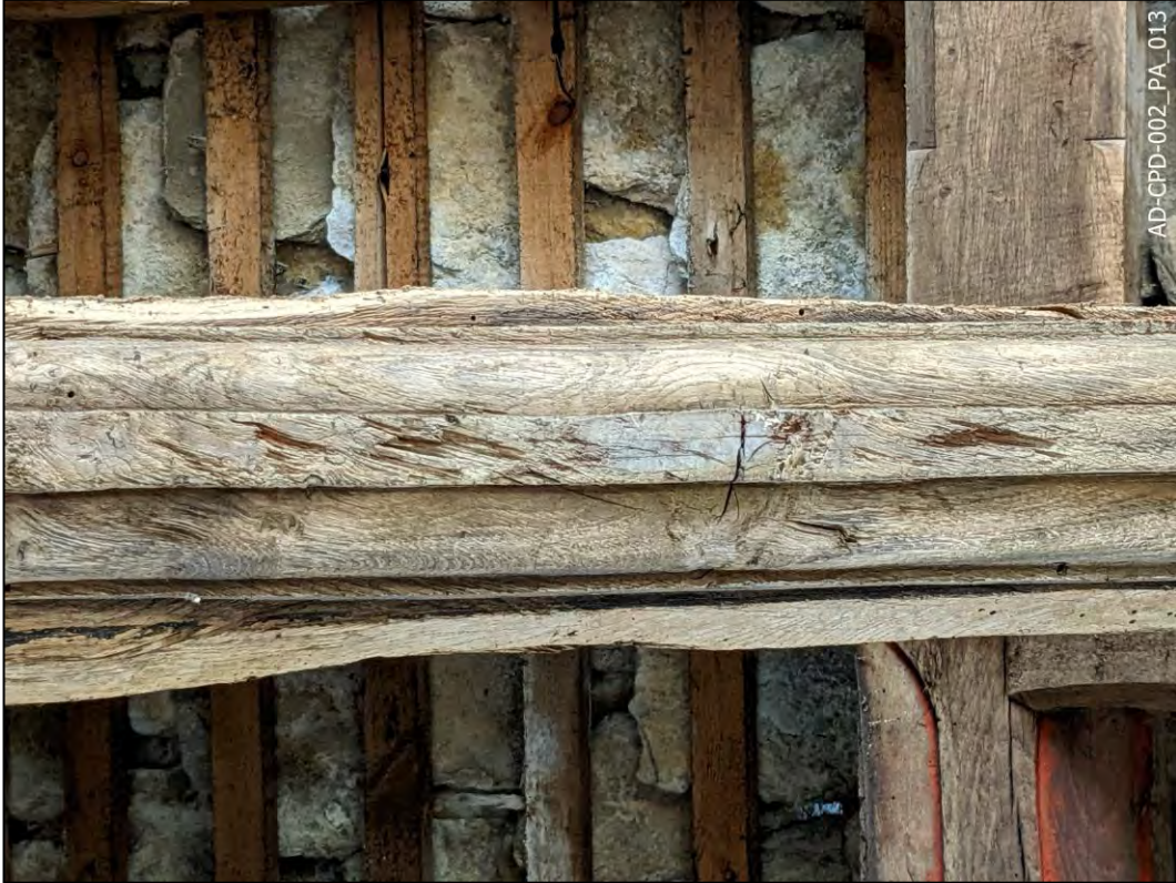
Plate 13 – Truss 8 – Arch-brace ovolo moulding – Rotated 90° anticlockwise
