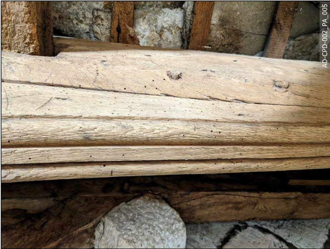
Plate 5 – Truss 1 – Arch-brace moulding – Rotated 90° anticlockwise
