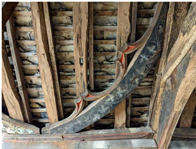
Fig. 7 – Typical wind brace detail.
