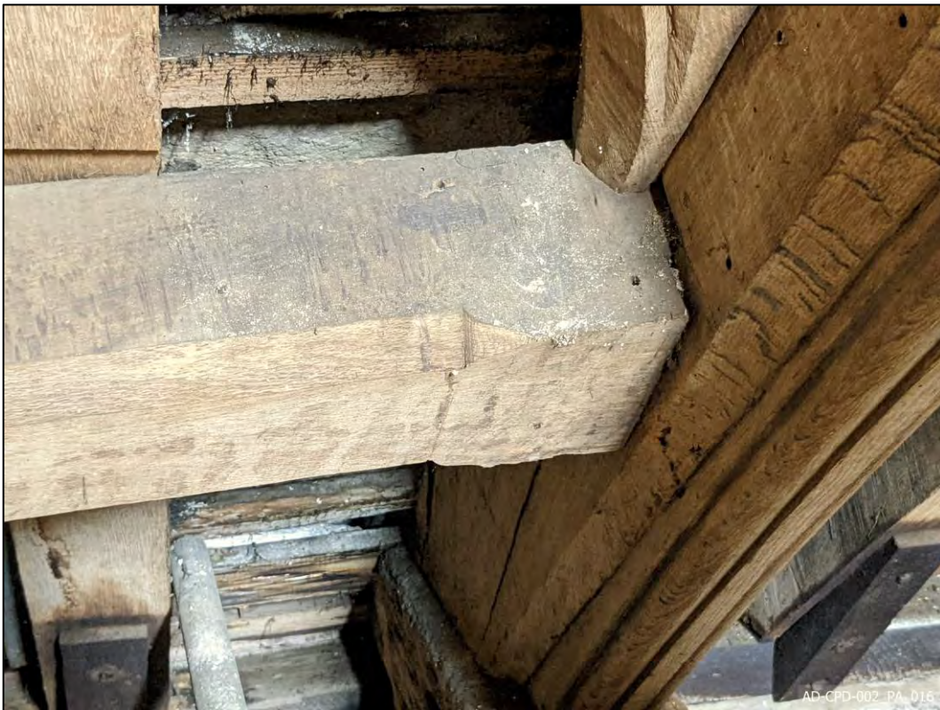
Plate 16 – General detail – Lower purlin
